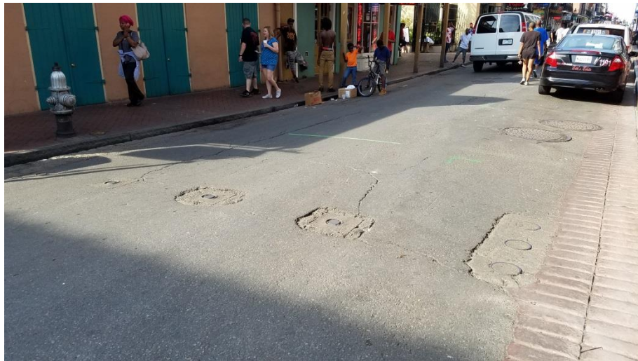
Figure 1 Existing Bourbon St Bollard Footings
