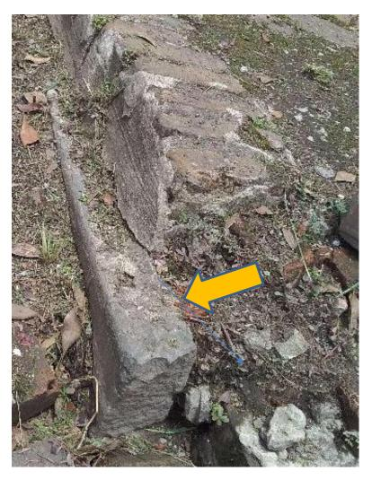
Figure C5. <u>Contributing status yet to be determined:</u> Brick Curb resting on top of bluestone curb (SEE ARROW), along 3000 block of Camp Street near catch basin, Garden District, NRHD/NHL, Period of Significance: 1832-1959
