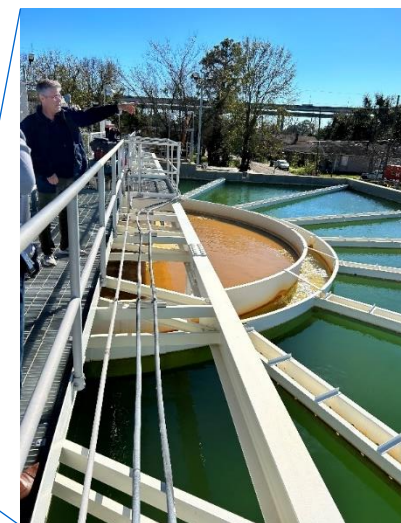
Algiers Water Treatment Plant
