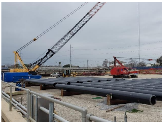
Power Complex Underway
