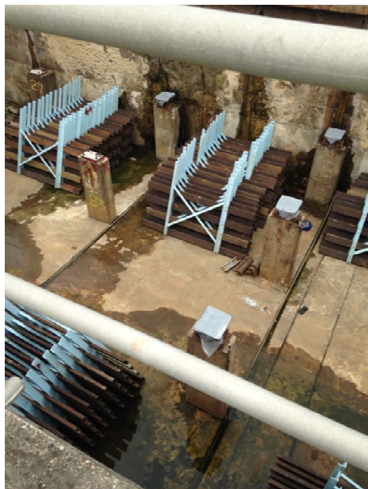
L3 Sedimentation Basin Flocculator Rehab
