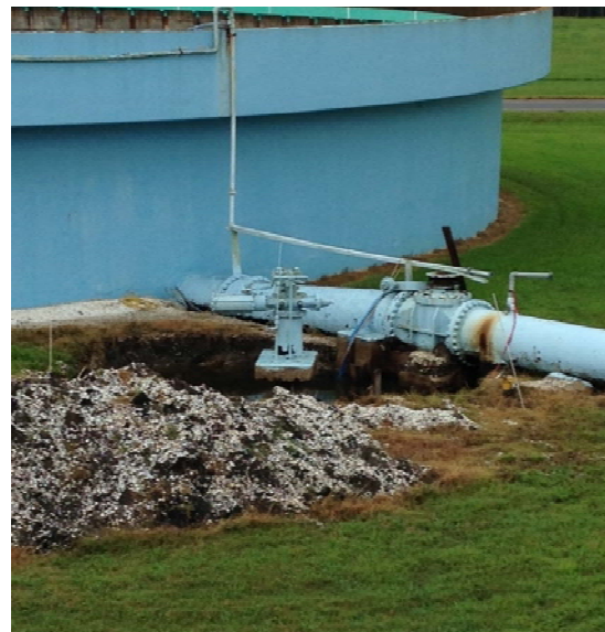
Valve repair on West Primary Clarifier in progress
