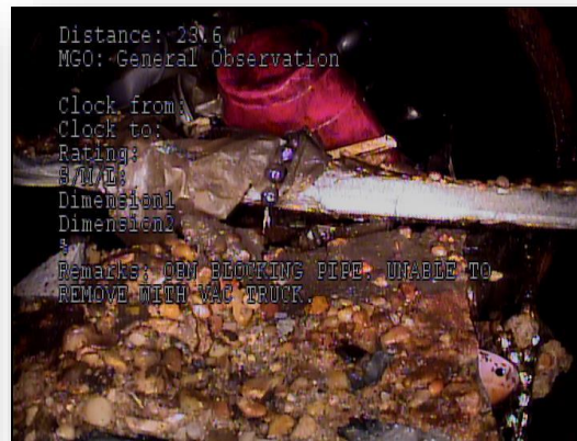
Debris filled, broken drain line between Orleans Ave. and St. Ann St.
