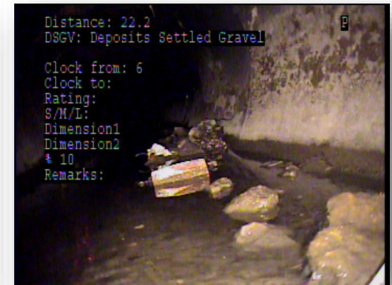
Fragments of a broken and undersized drain line between Iberville and Bienville streets.
