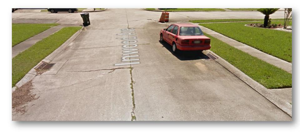
Existing condition 4000 block of S. Inwood Ave. – Pavement Condition Index - Very Poor
