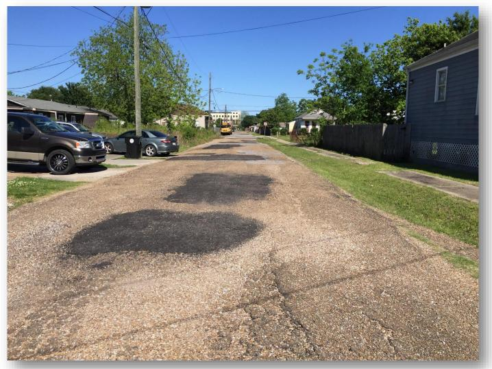
Existing condition 1300 block of Evelina St. – Pavement Condition Index - Very Poor
