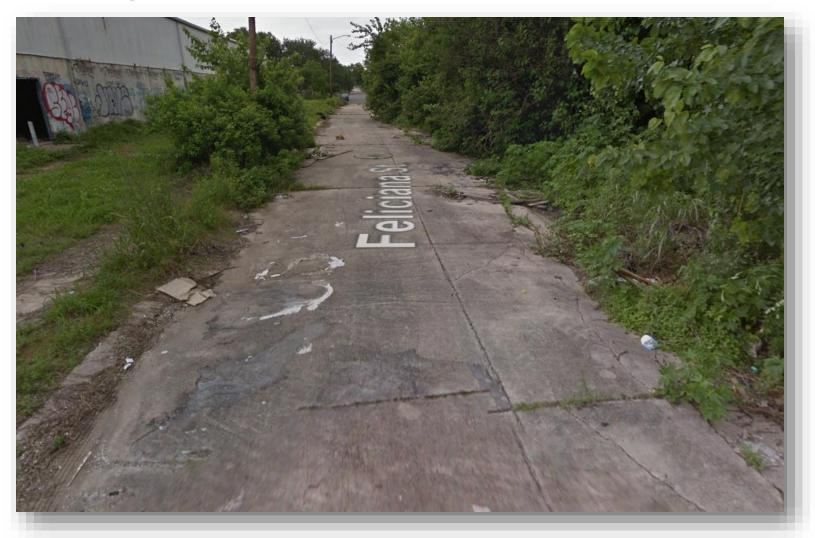
Existing condition 2800 block of Feliciana St. – Pavement Condition Index - Very Poor
