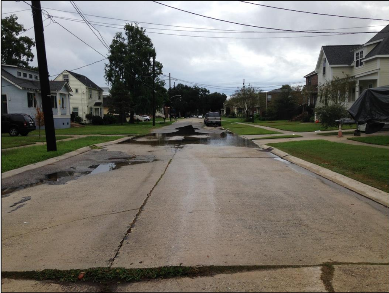
Existing condition of the 6800 block of Catina St. in Nov. 2015.
