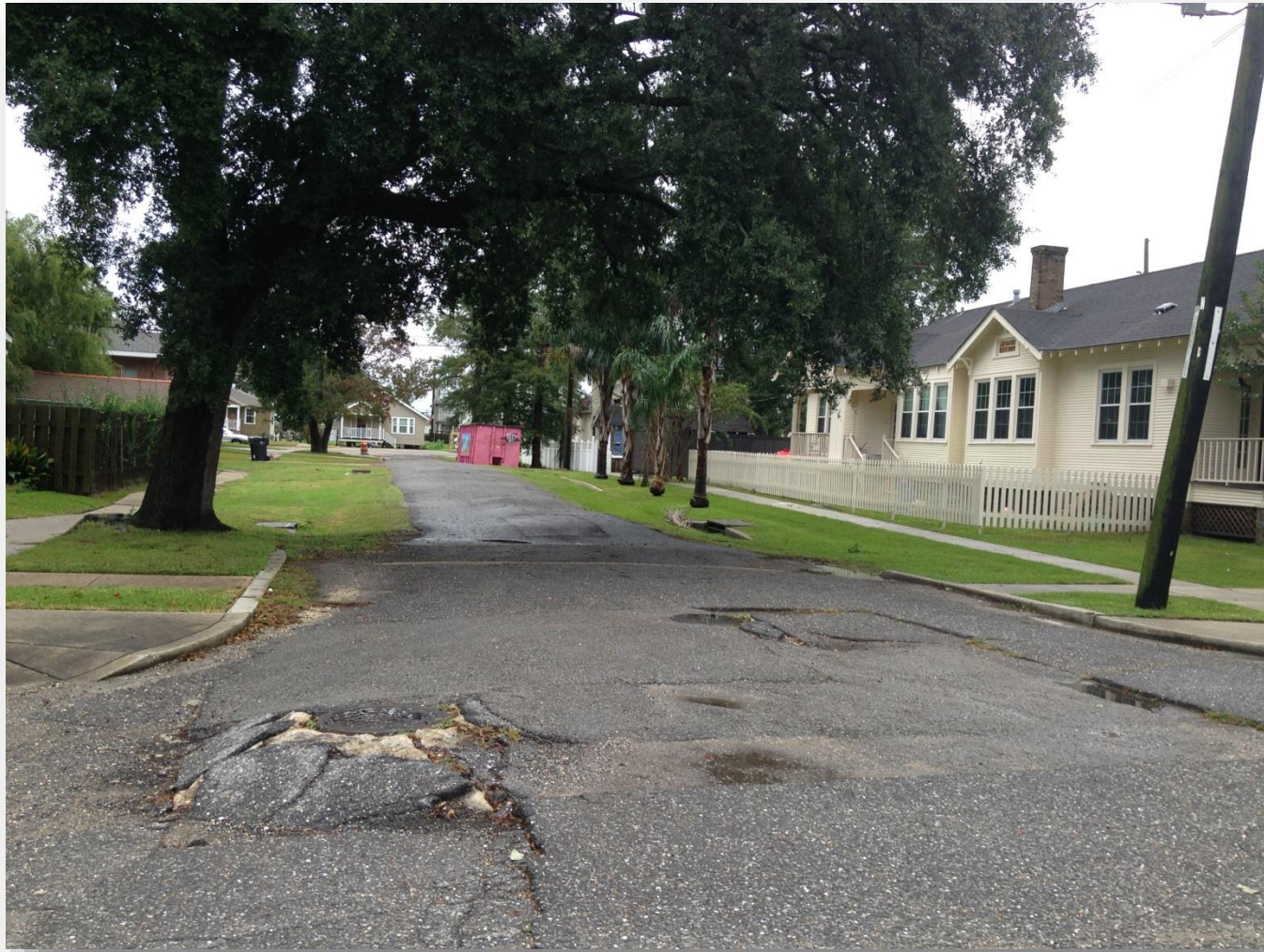
Existing condition of the 200 block of Fremont St. in Nov. 2015.
