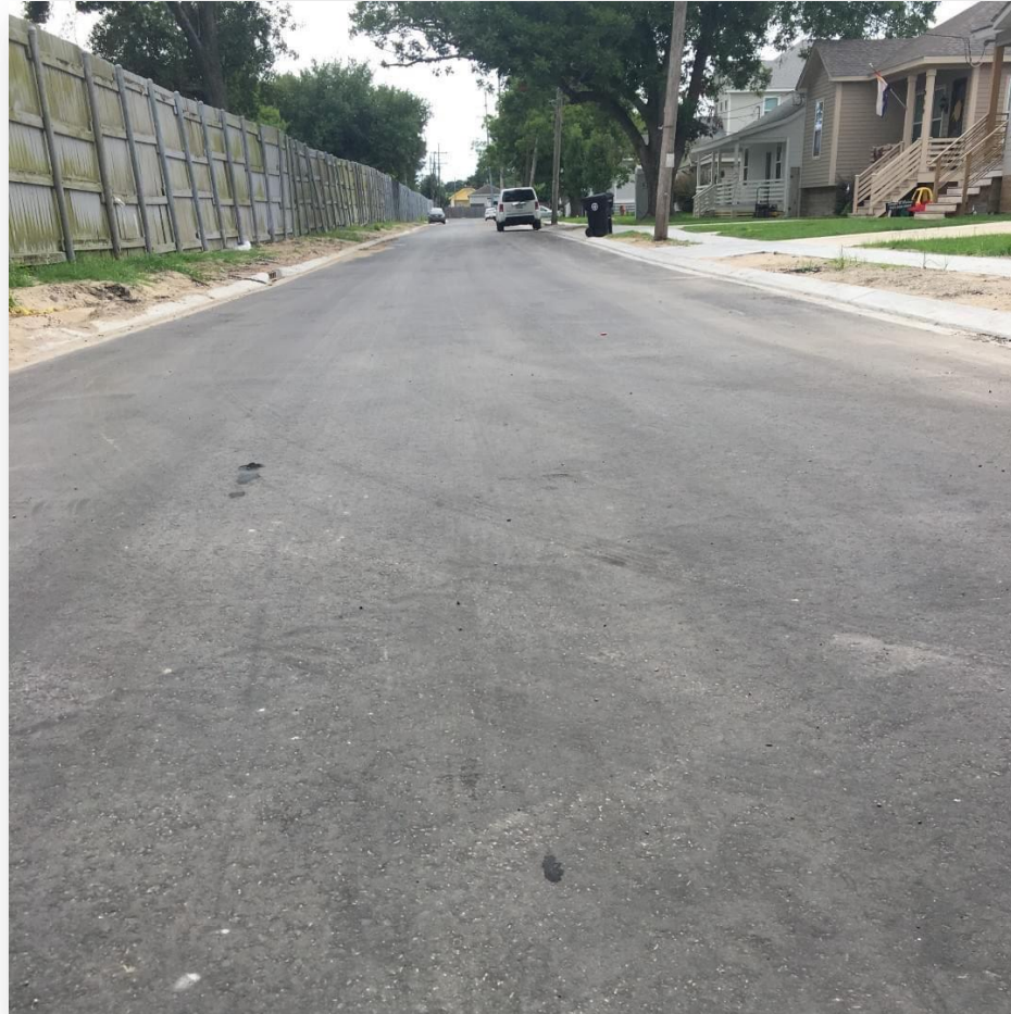
An example of a repaved area of Kenilworth St. from the recently completed Lakeview South Group A.
