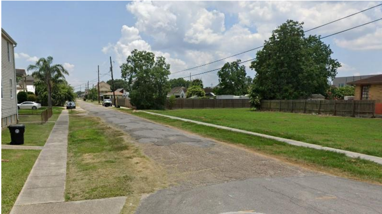
Existing conditions on the 2300 block of Vienna Street
