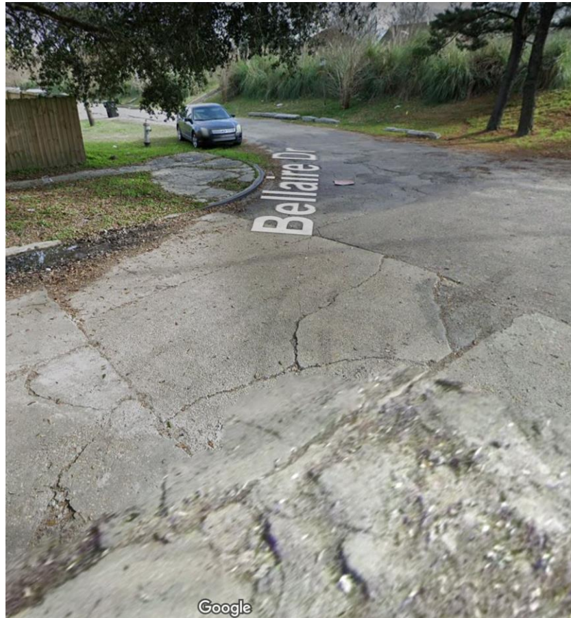
Existing condition of the 6000 Bellaire Dr.
