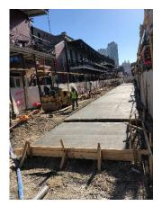
The new waterline and drain line have been completed. The new concrete roadway is being poured today (pictured). Crews will be removing the fence and installing granite curbs this weekend. Roadway work (not sidewalk work) in this section of the 700 block is anticipated to complete by February 18.
