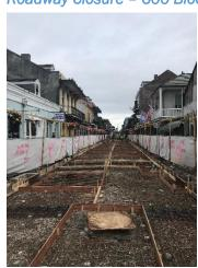
Crews have completed work on the new waterline and new drain line. Crews are continuing to prepare for concrete pours next week (pictured). Currently, the 600 block is scheduled to reopen to pedestrian traffic on or before January 27, weather permitting.
