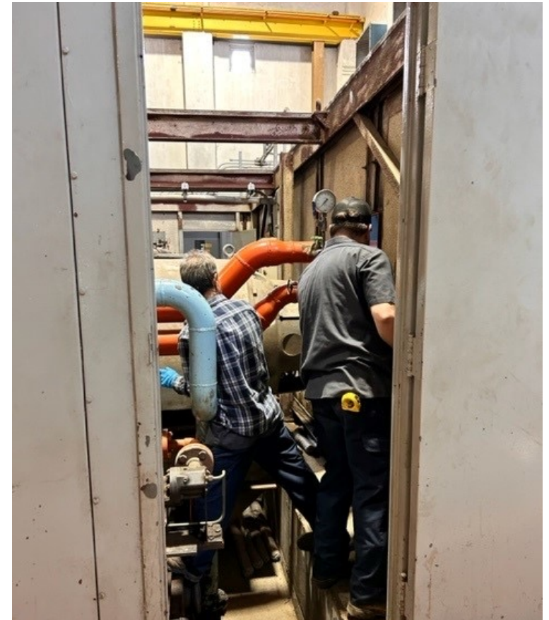
Work happening on Turbine 5, Dec. 5
