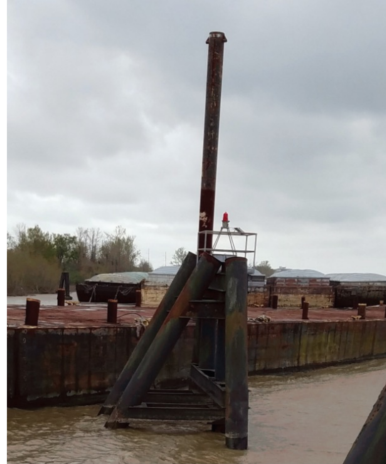
Additional Pictures of Damaged Intake Fender System and Temporary Barge
