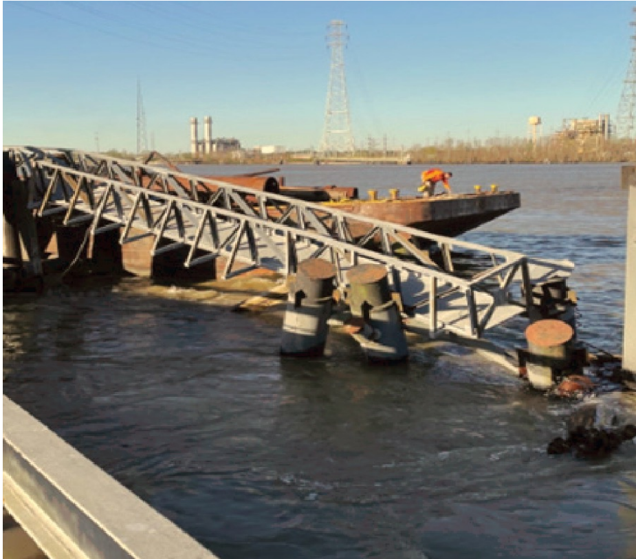
Additional Pictures of Damaged Intake Fender System and Temporary Barge
