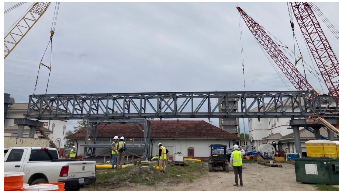
Span 29 installed on 3/21/2024
