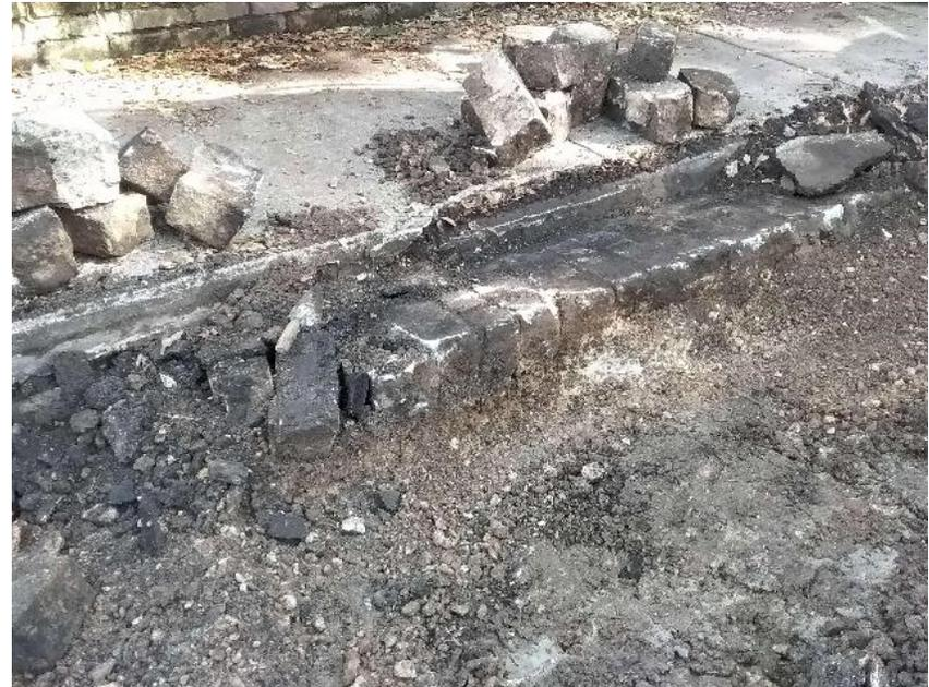
*Figure 3. Granite pavers discovered beneath asphalt at Garfield Street between Octavia and Arabella.*
