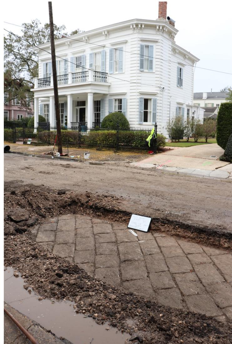
*Figure 4. Large granite pavers discovered beneath asphalt at First St. and Prytania St. in the Garden District.*
