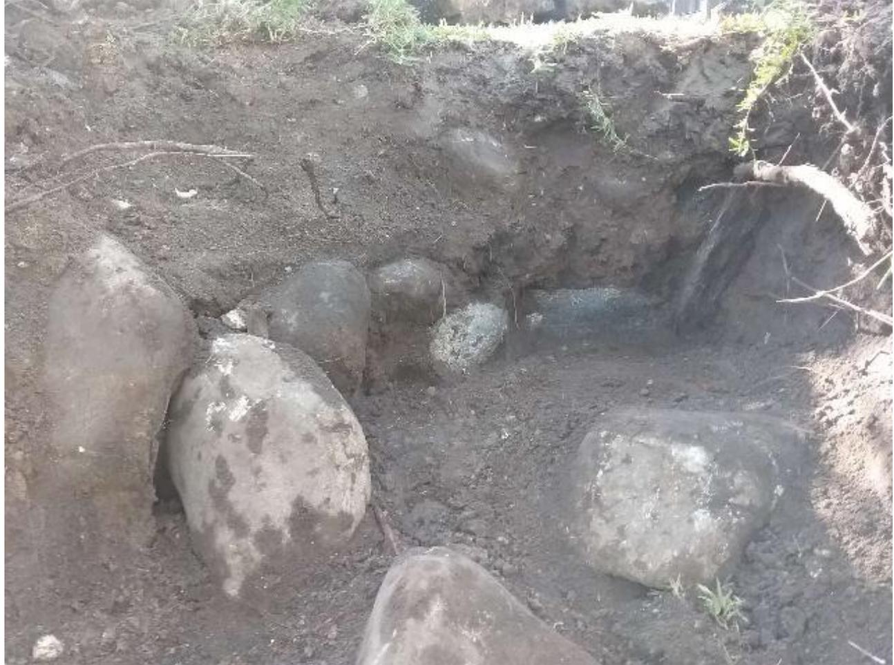
*Figure 4. In situ granite curb at 75 degree angle next to cobblestones observed along Bayou Road.*
