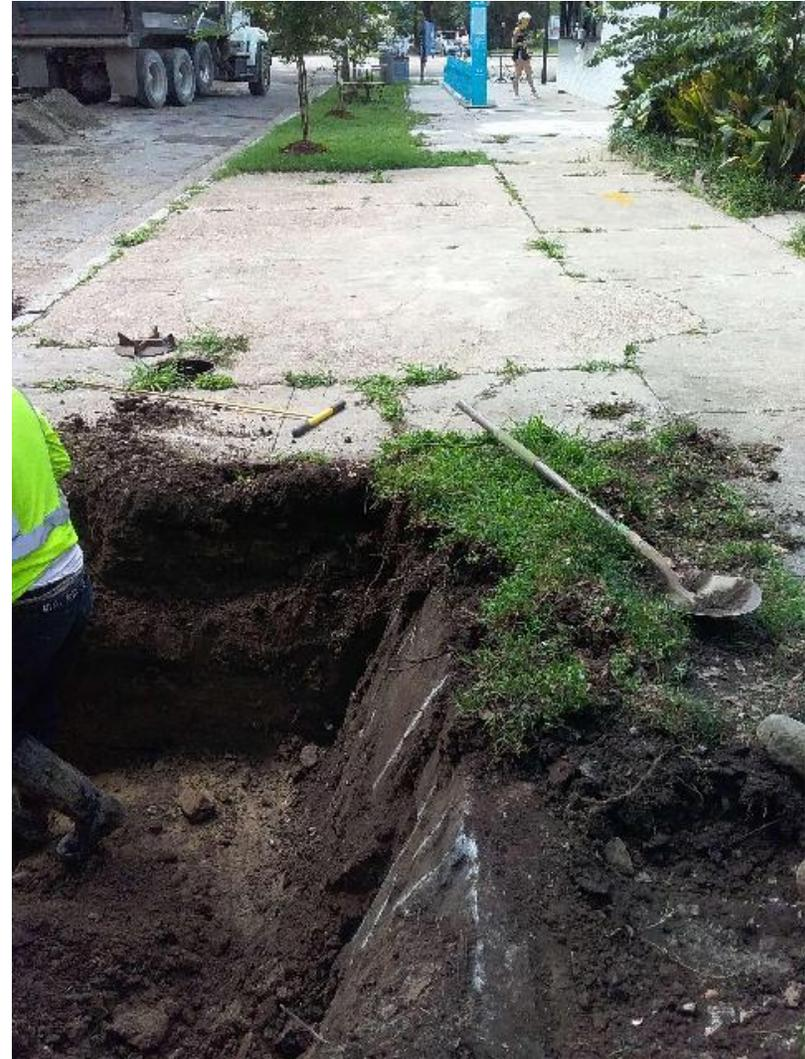
*Figure 5. Granite curb with modifications to allow for house connections; curb continues to the end of the street.*
