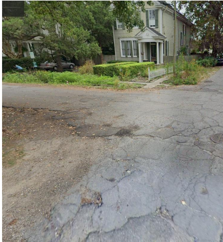
Existing conditions on the 300 block of Millaudon Street
