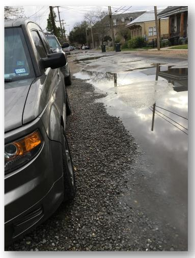
Uneven pavement and lack of drainage causes water to pool during rain events.
