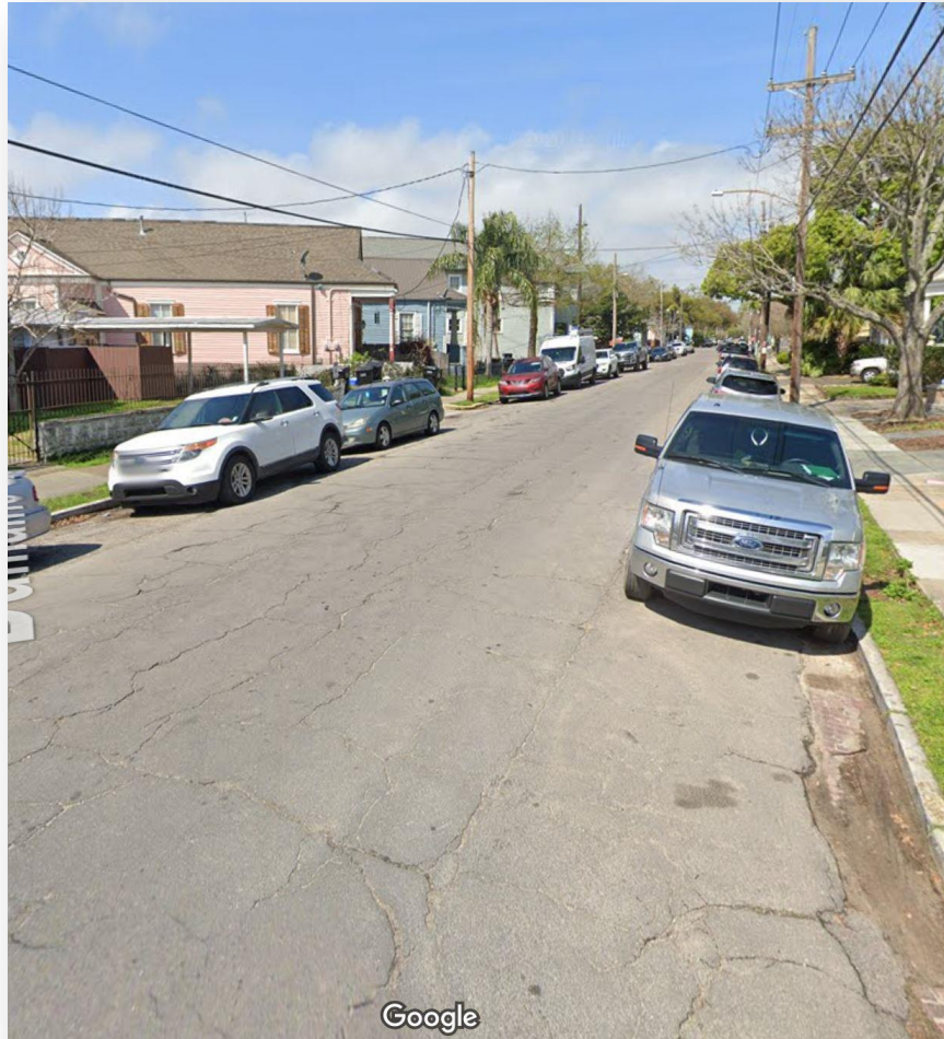
Existing condition of 3600 block of Dumaine Street.
