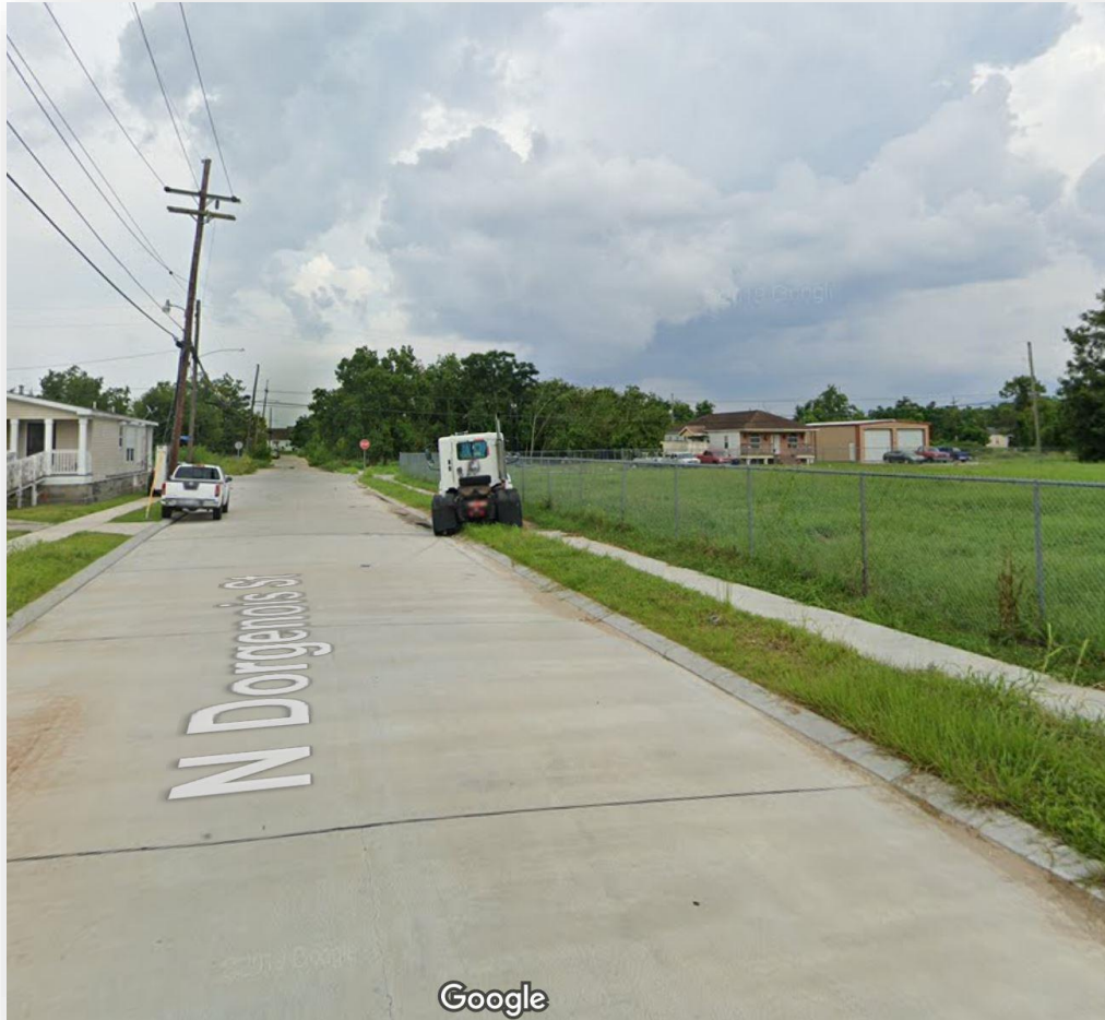
An example of a repaved area of N. Dorgenois St. from the recently completed Lower Ninth Ward Northeast Group A Project.
