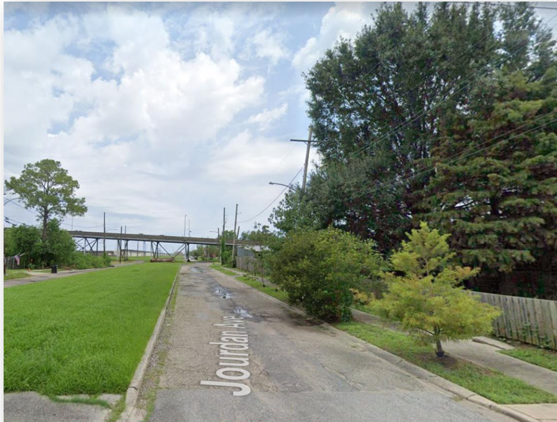
Existing condition of Jourdan Avenue at S. Robertson Street.
