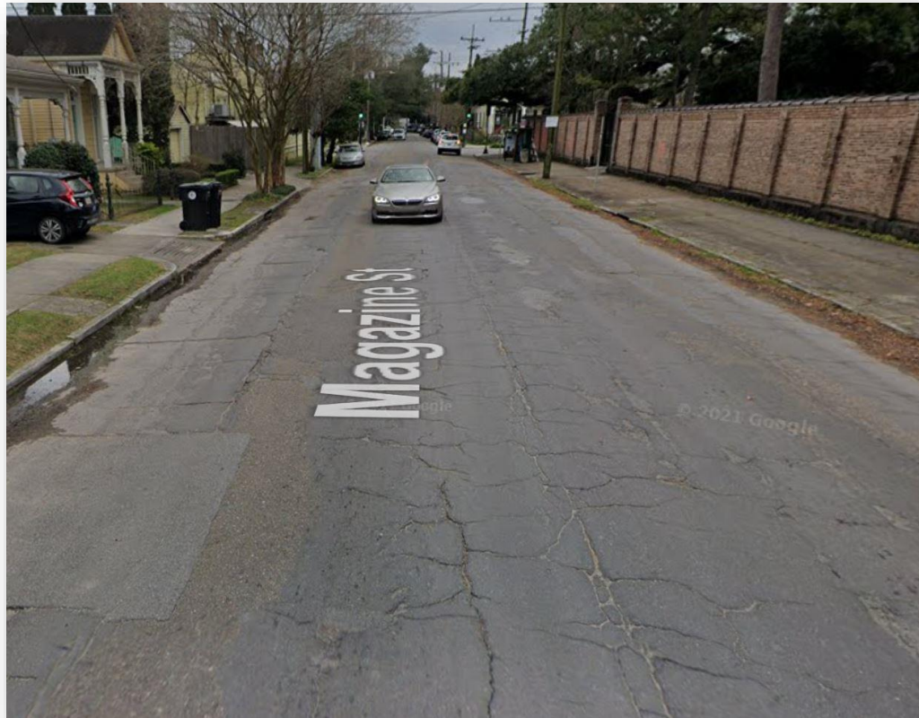
Existing asphalt conditions on the 6300 block of Magazine Street
