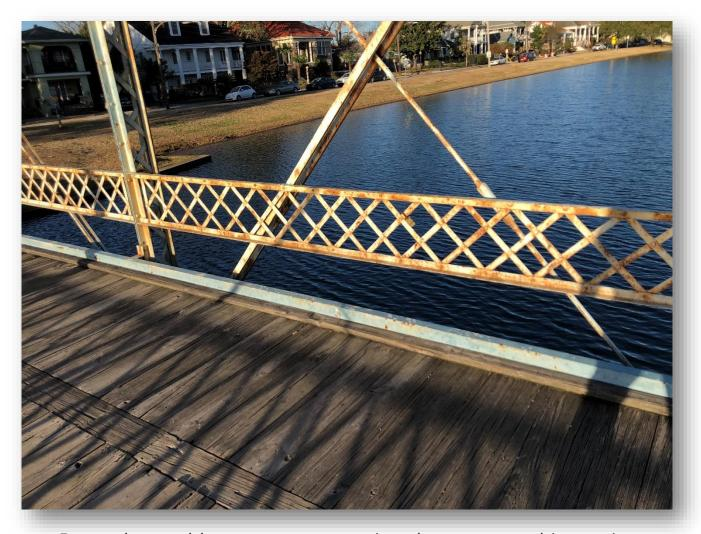
Rusted metal beams compromise the structural integrity
