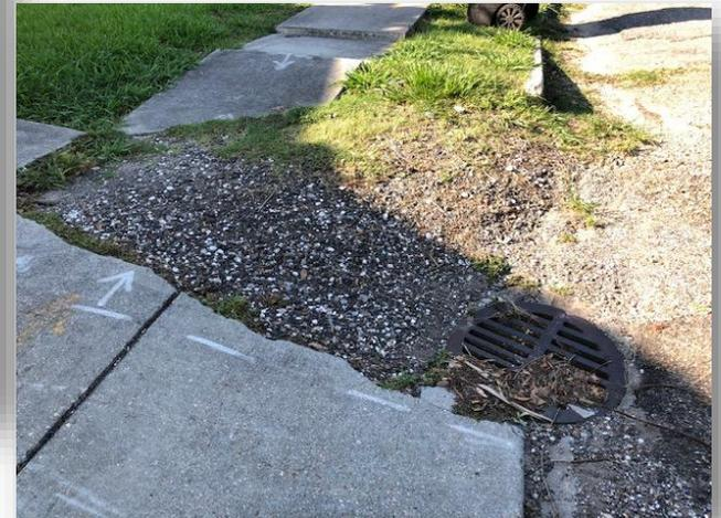
**Existing conditions on Taft Place. Pavement Condition Index is Failure.**
